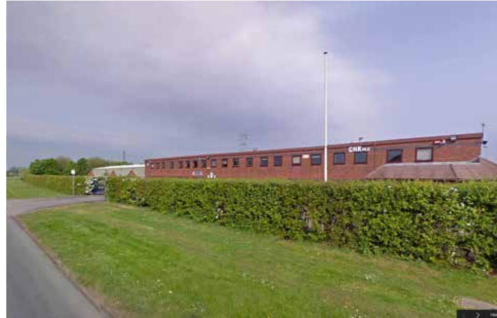
CHK Building on Pyms Lane
